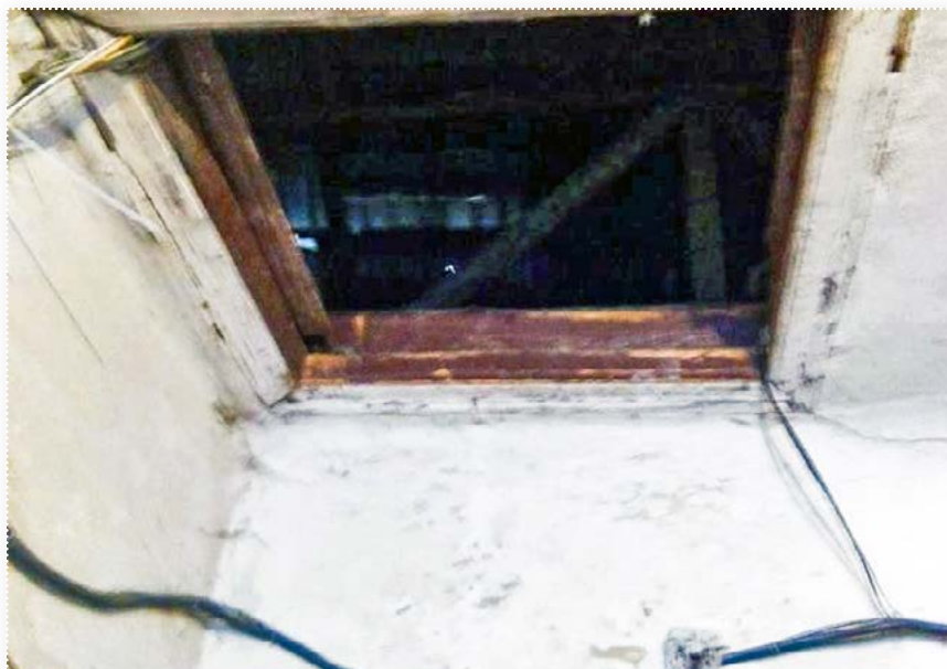
Entrance to the attic of the house No.381
