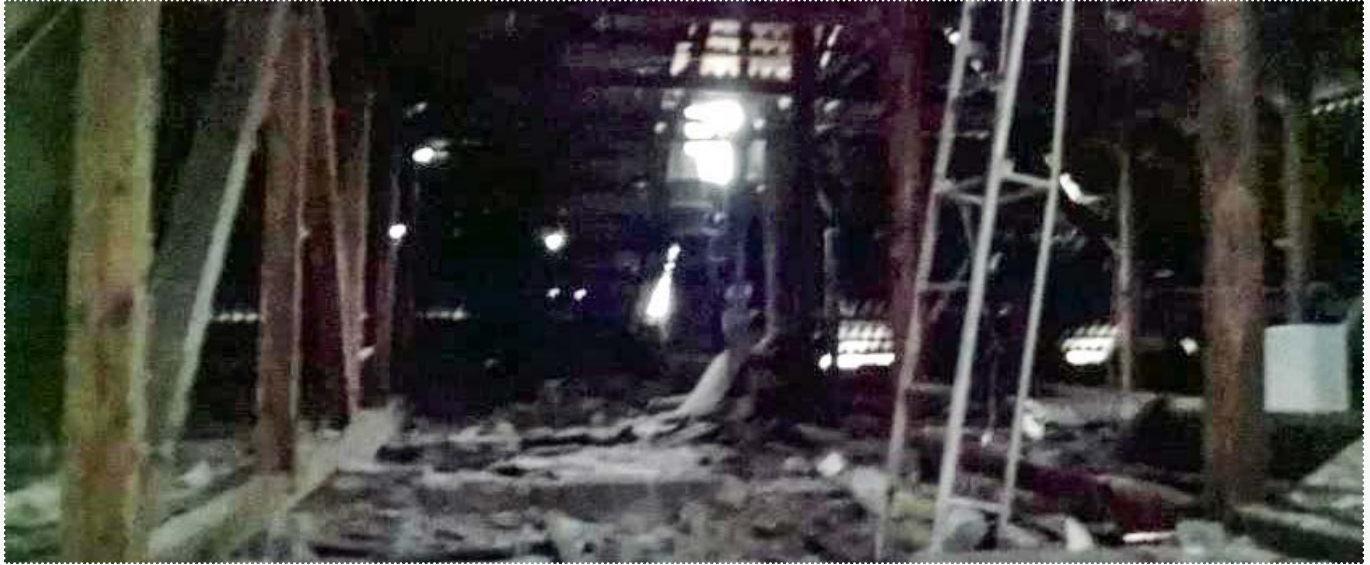
The attic of the house No.381
