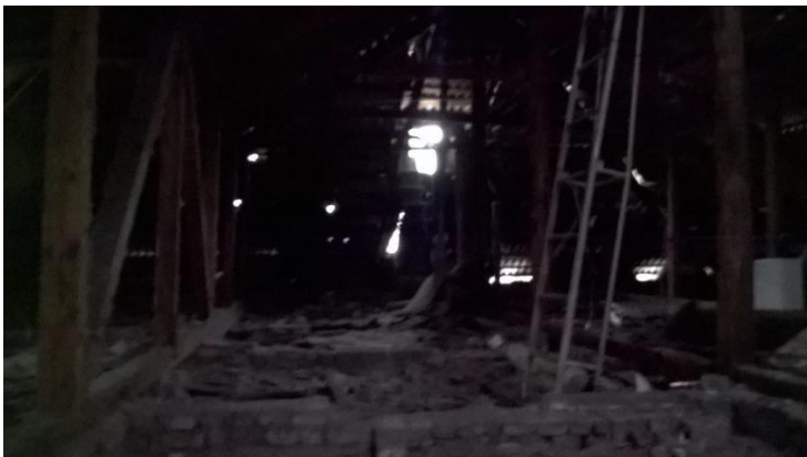
The attic of the house No.381
