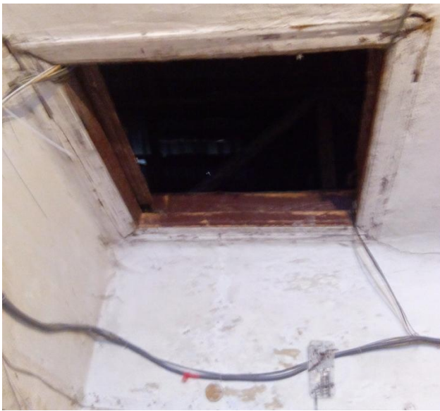
Entrance to the attic of the house No.381
